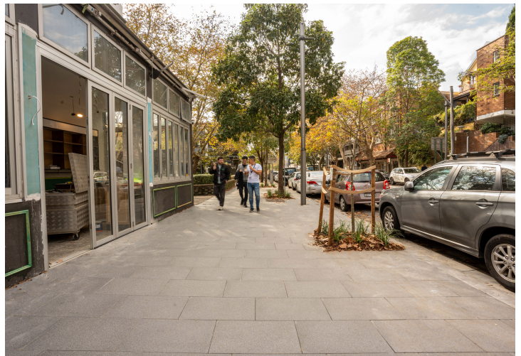
Above: completed works south of Reservoir Street in May.
